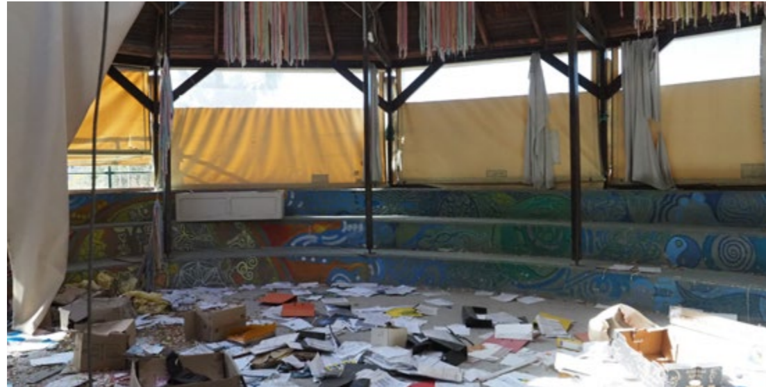
Scattered documents in the ruins of the events hall at Karatepe reception facility in Lesbos after it was abandoned © Olga Demetriou, October 2022
